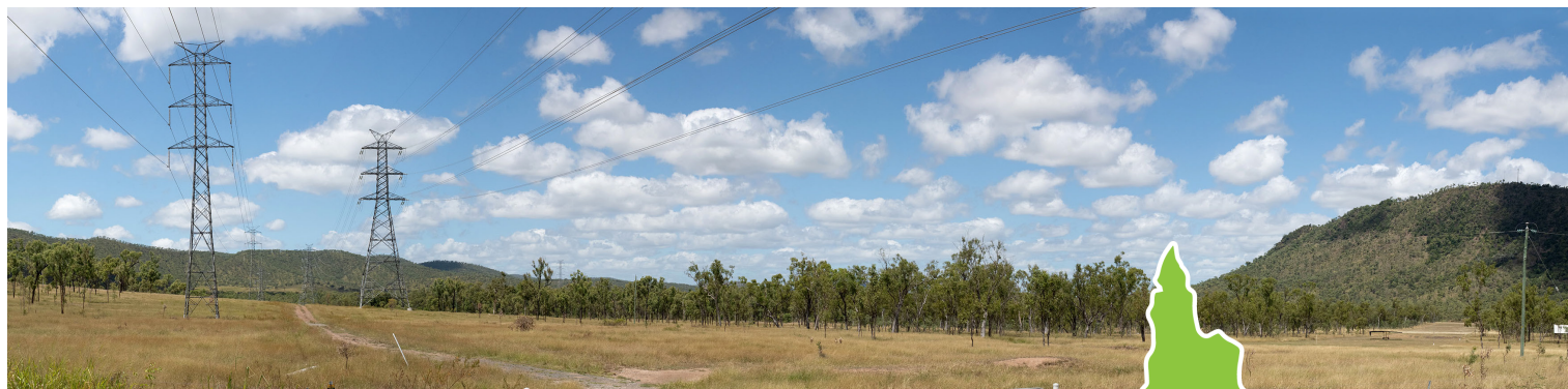
Photograph of the project area
