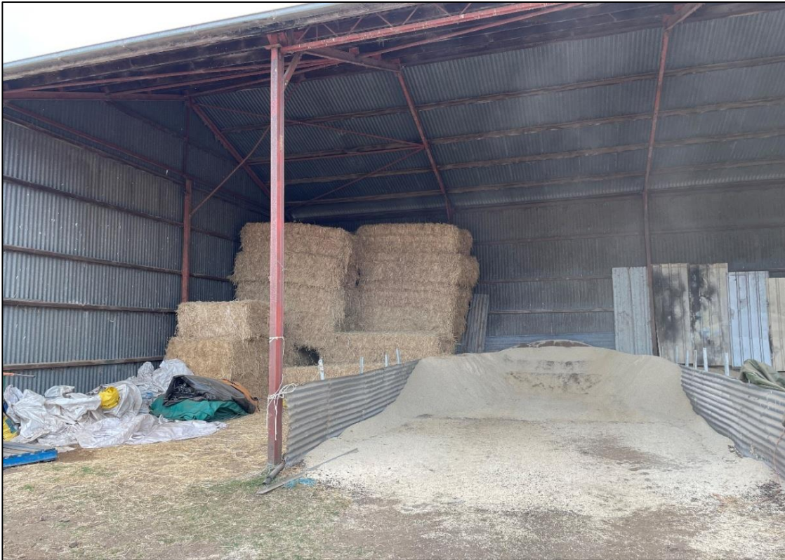
Plate 6: Chemicals and fertilisers were observed to be appropriately stored in designated areas outside of the amended Development Footprint.
