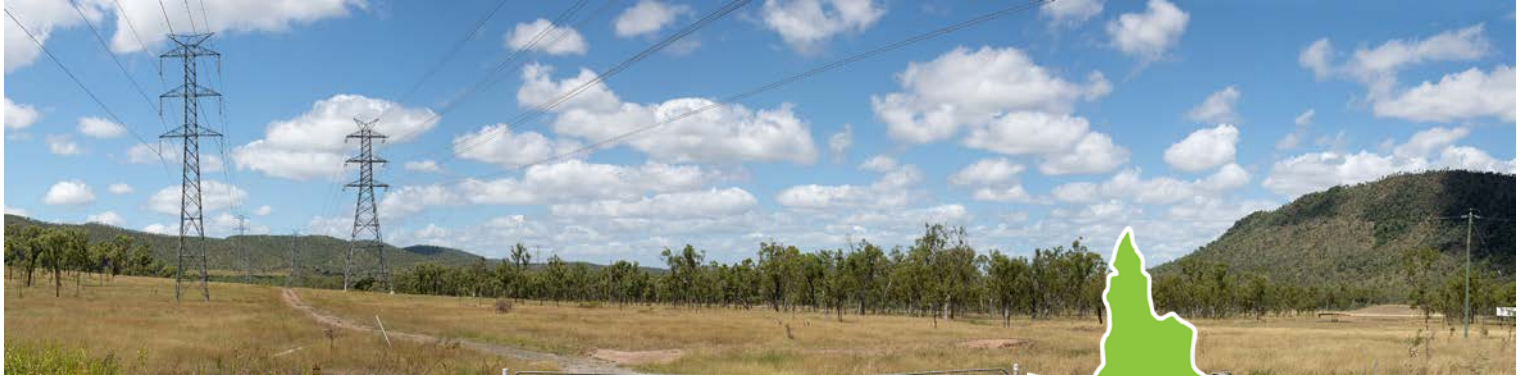
Photograph of the project area
