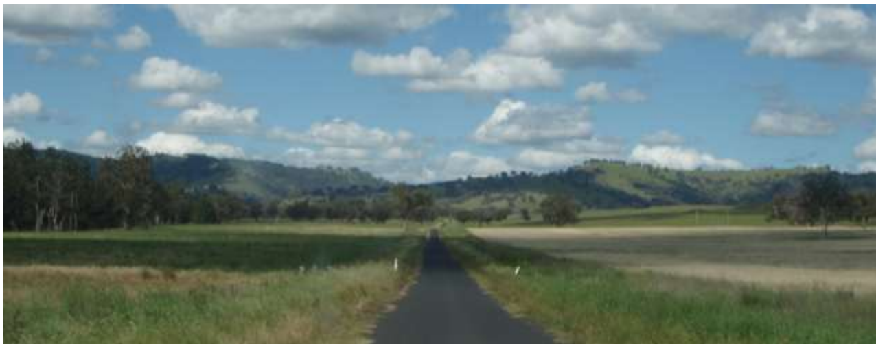
View east along Coolah Creek Road
