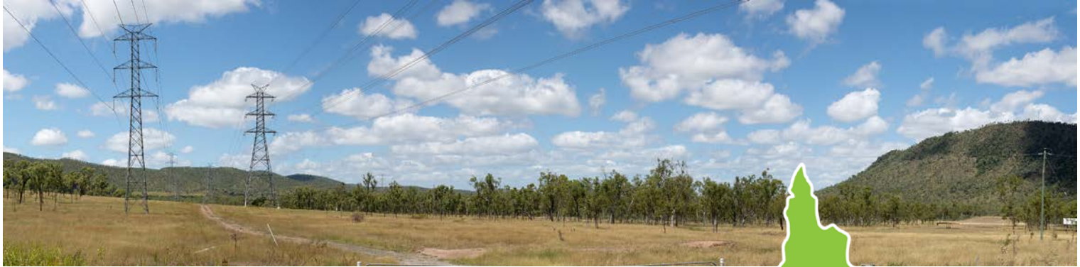
Photograph of the project area
