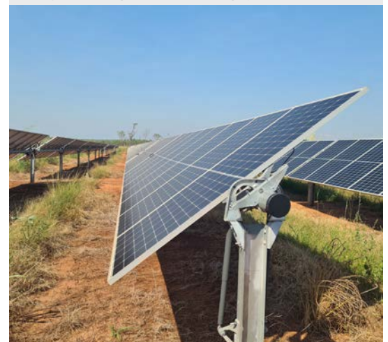
Example of a single axis tracking system
