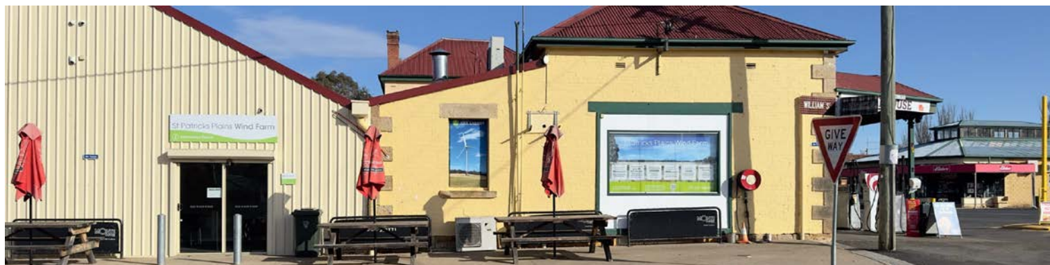
St Patricks Plains Wind Farm Information Centre in Bothwell
