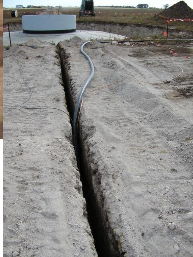
Cable trenching (underground cabling)
