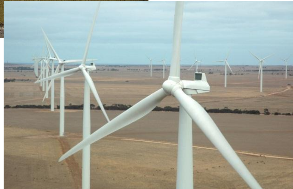
Completed wind farm
