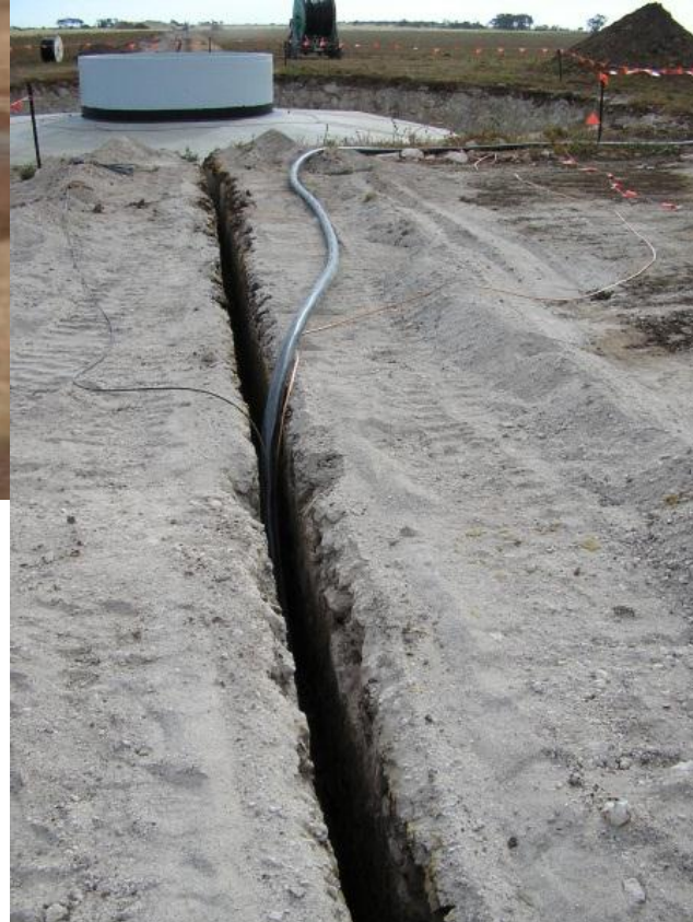
Cable trenching (underground cabling)
