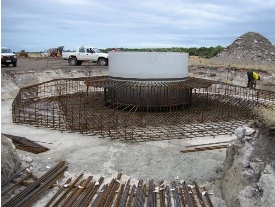
Foundation steel reinforcing
