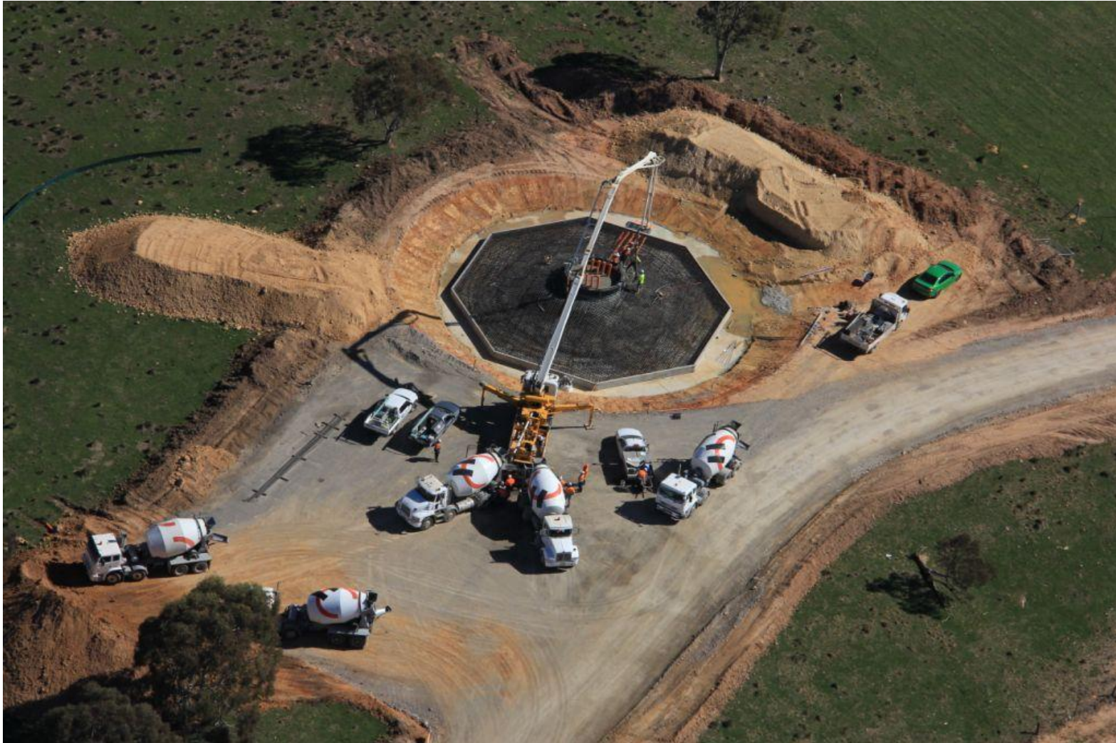
Foundation under construction
