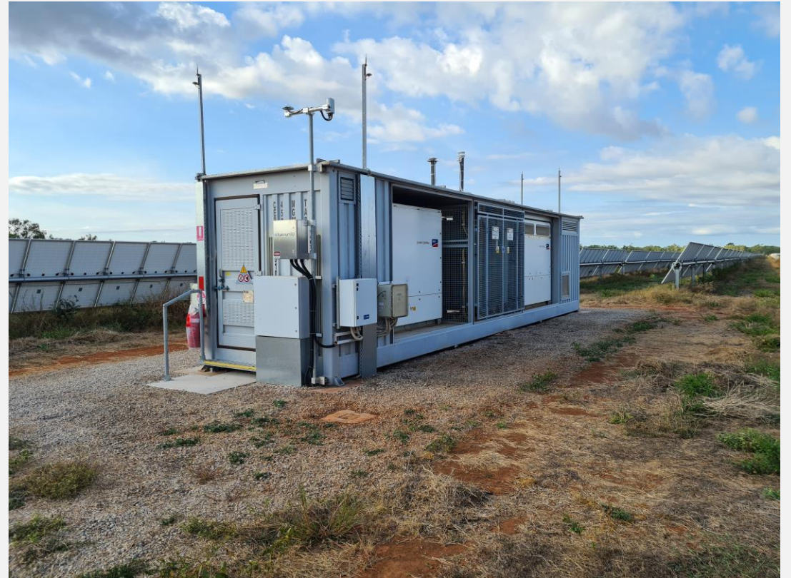
Inverter – Converts direct current (DC) electricity to alternating current (AC) electricity
