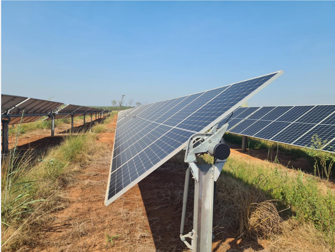
Solar Panels - Single Axis Tracking
