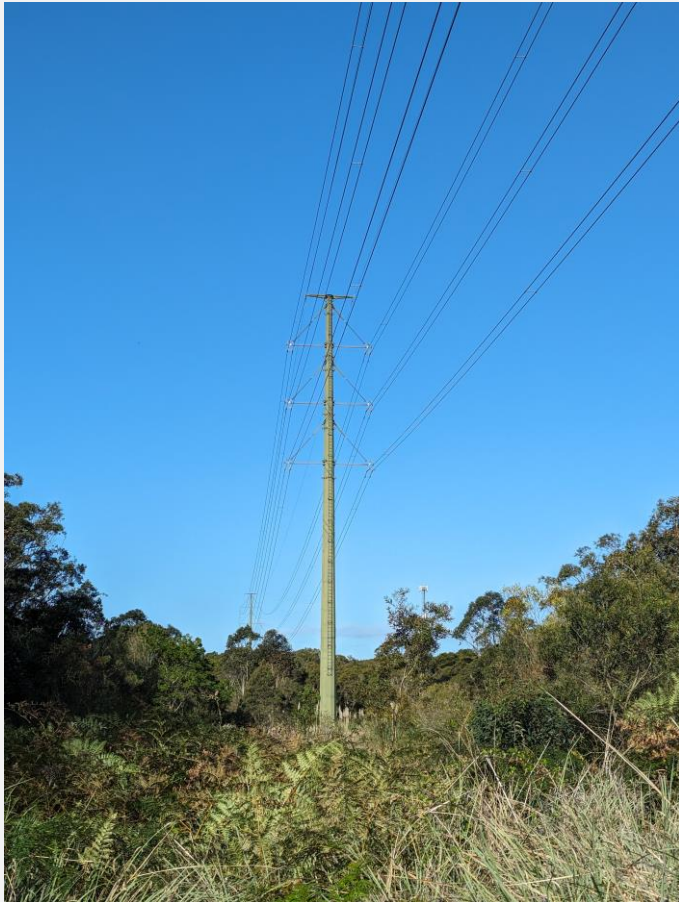
Transmission Lines – 330kV 60m single pole construction
