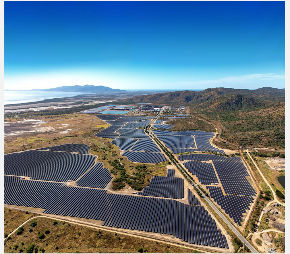
Sun Metals Solar Farm
