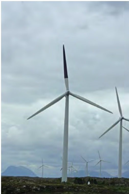
Figure 6-9 Example of black painted WTG blade used to decrease motion blur (May, et al., 2020)
