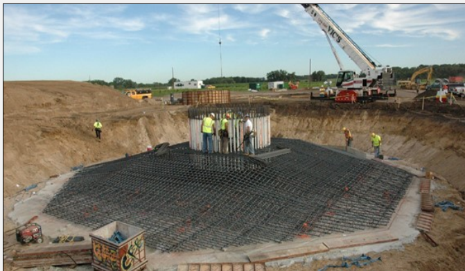
Tower foundations ~800m 3 concrete.
