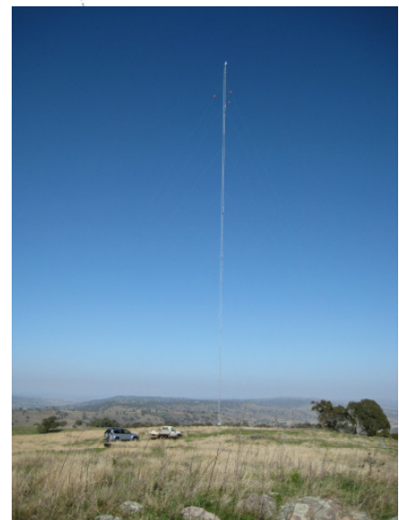
Figure 2 Mast onsite at Liverpool Range
