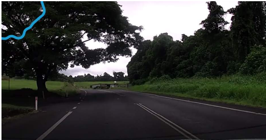
Figure B1 – Example of required pruning from overhanging tree branches, located on Palmerston Highway, 13.7 km from Bruce Highway
