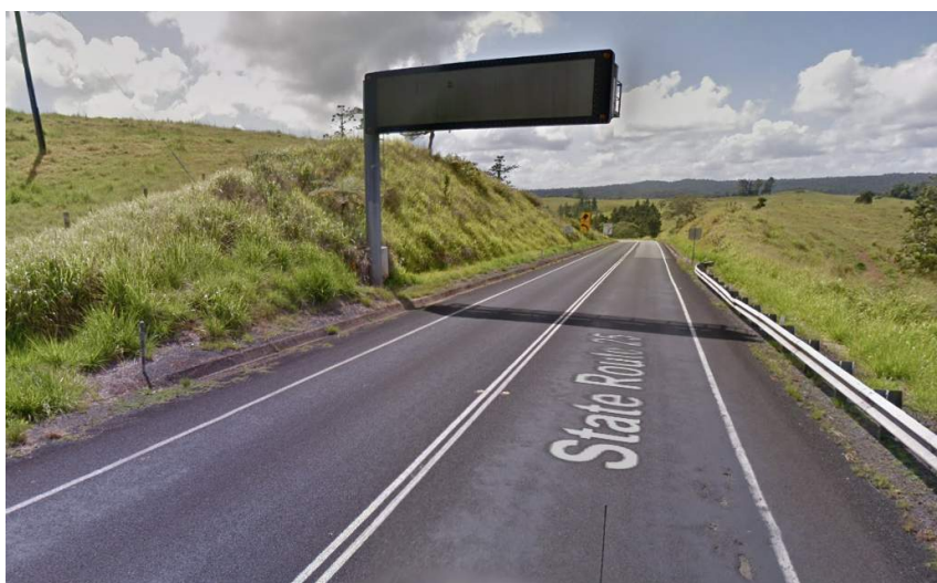
Figure B3 – Overhead Electrical Road Sign
