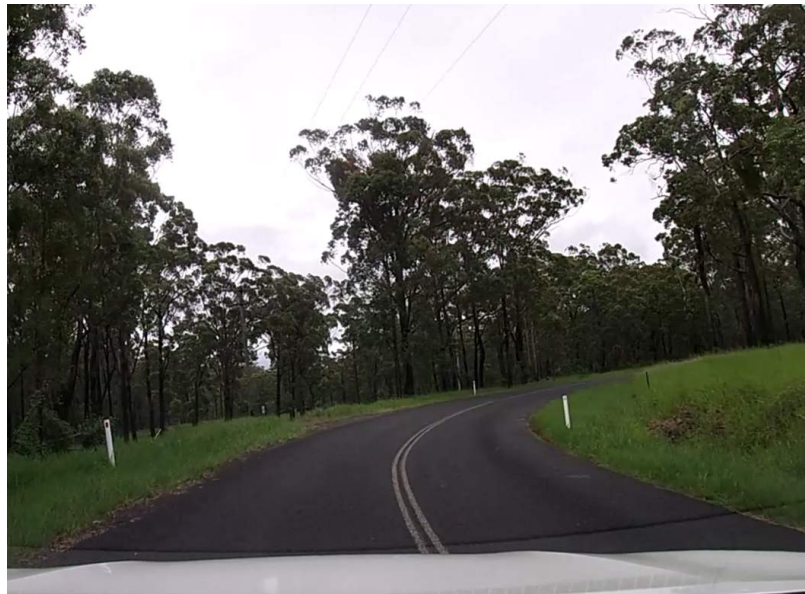
Figure 11 – Wooroora Road Overhead Lines
