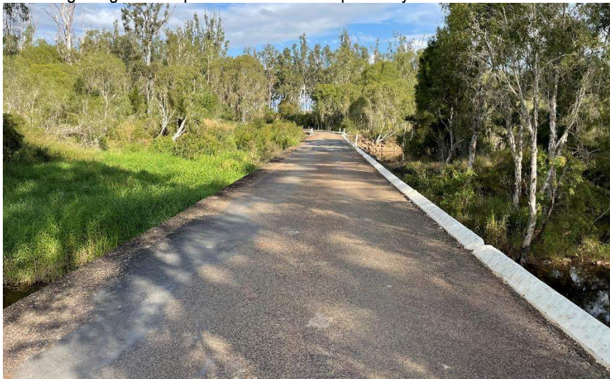
Figure 14 – Herbert River Bridge (12 th September 2022, looking south)
